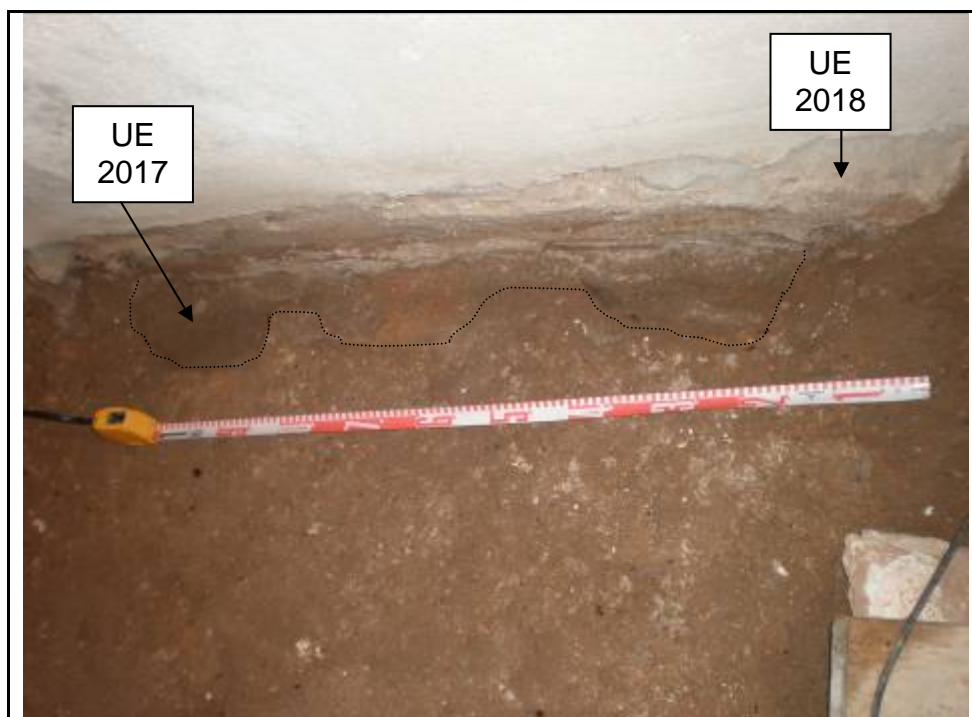
41. Rasa 2017 i mur 2018
